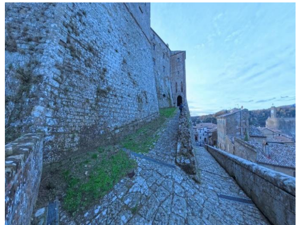
71 last stretch of the two steep and irregular ramps that lead to the village level
