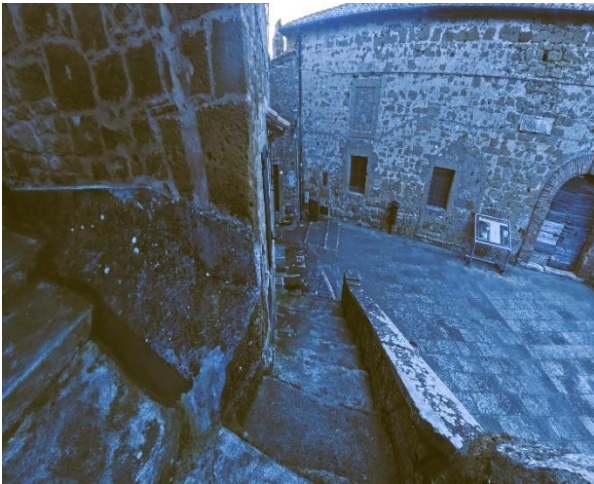
48 Stairways to reach the Leopoldino Keep
