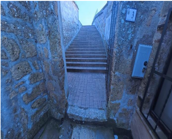
50 stairways to reach the Leopoldino Keep
