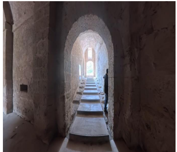
59 Second access door with steps
